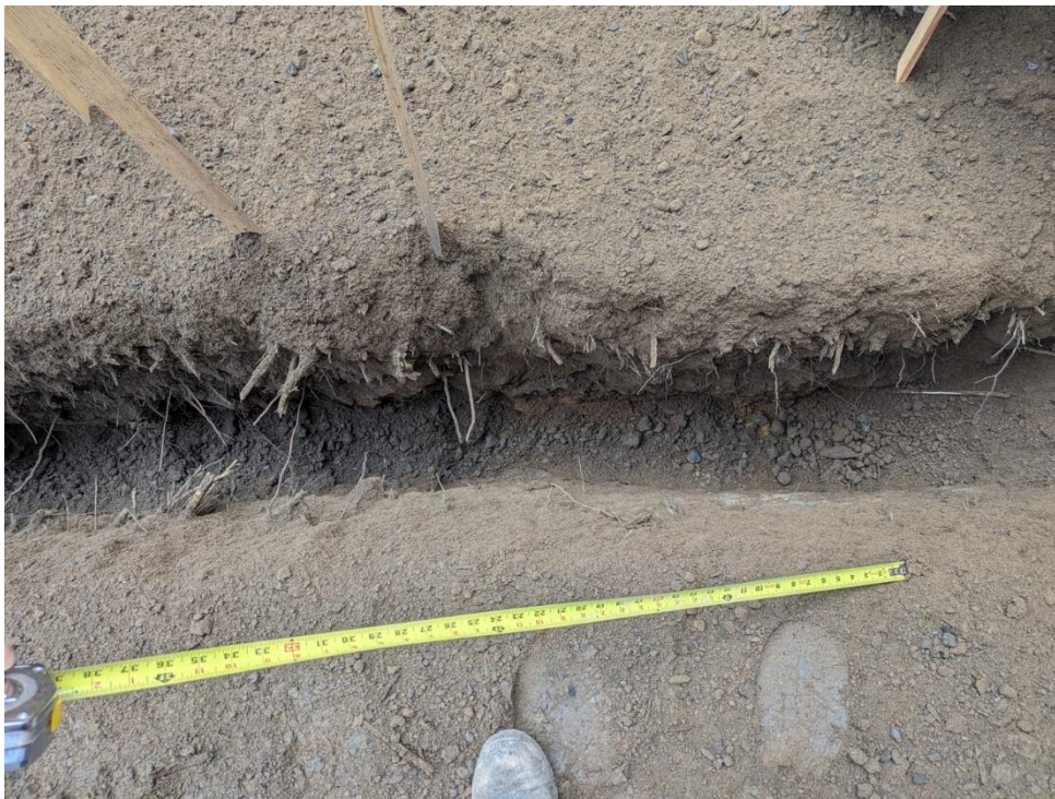
Photo 3. A typical section of trench with small feeder roots are exposed.
