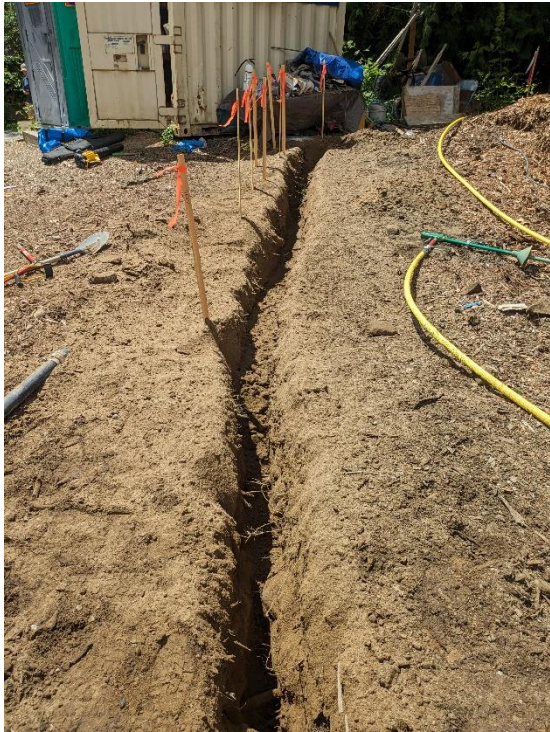
Photo 2. View of the trench from the north following pneumatic excavation.
